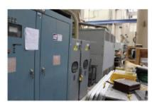
In addition to various bench top instrumentation power supplies, CEM also has a 250 Volt 6,000 Amp dc power supply located in the main high bay. 4160 V available in the second story transformer vault, with 480 V available throughout the high bay.
